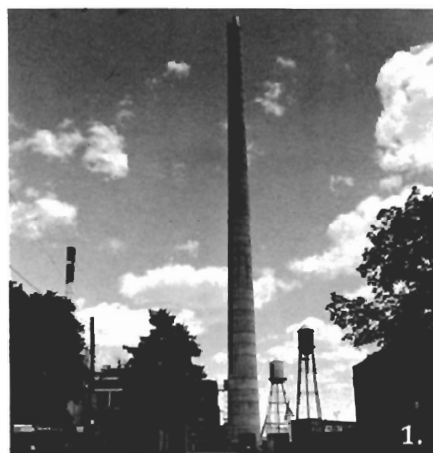
1. Concrete stack with dual flues to ensure air quality, St. Lawrence Starch Company Limited, Port Credit. 2. Chilled water plant, University of Toronto. 3. Hydroelectric power development, Nam Ngum, Laos. 4. Underground powerhouse, Churchill Falls
