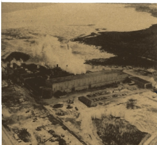
Fort William Division expansion shows paper machine room, finishing room and shipping warehouse in centre of picture, and expanded woodroom facilities on extreme left.
