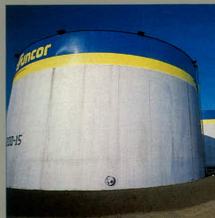
Storage tanks for synthetic crude oil.
