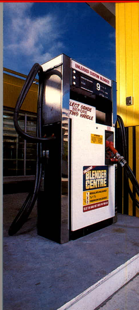
This Blender Centre pump provides three blends of unleaded gasoline. Its counterpart dispenses as many blends of leaded gasoline.
