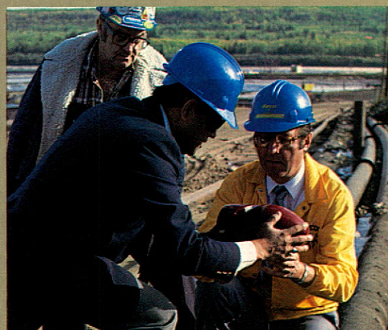
Bullet-like polyurethane "pigs" like this one clean internal corrosion to improve flow in underground water pipes at the oil sands plant.
