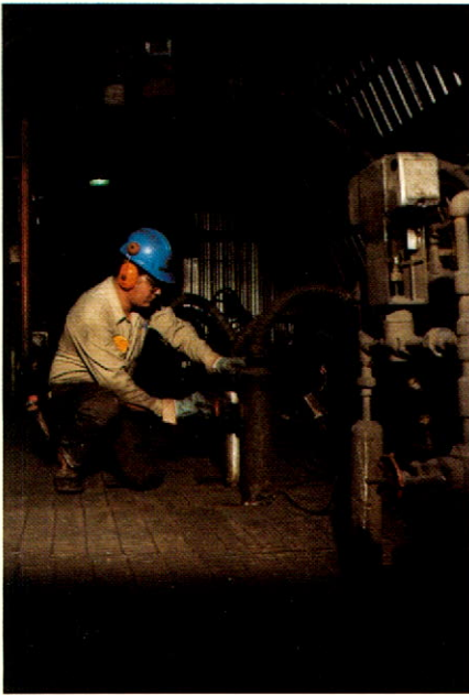
Len Maraschuk checks fuel supply to the powerhouse furnace at Suncor's oil sands plant.
