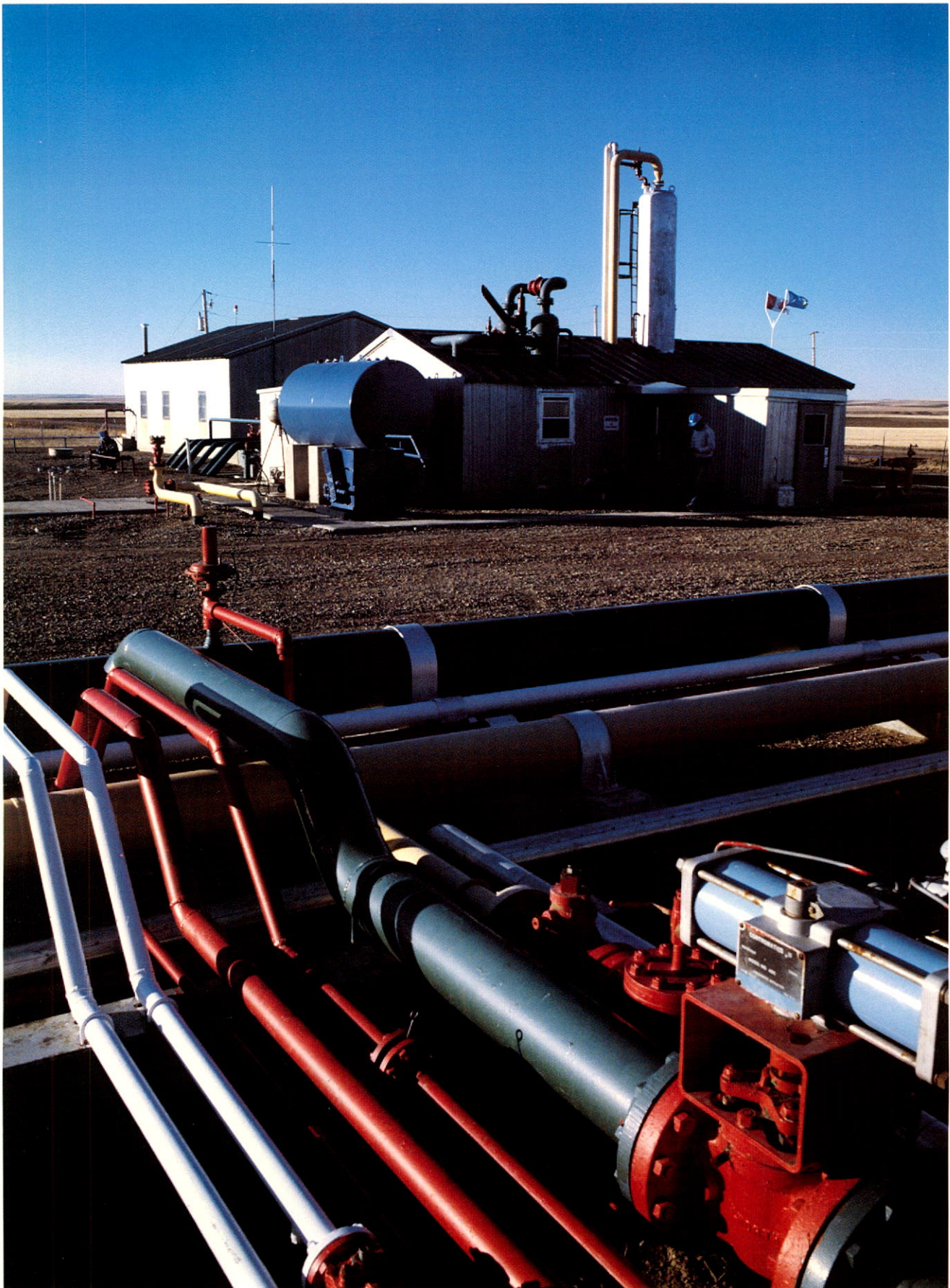
Natural gas compressor facilities capable of producing 18 mmcf/d.
