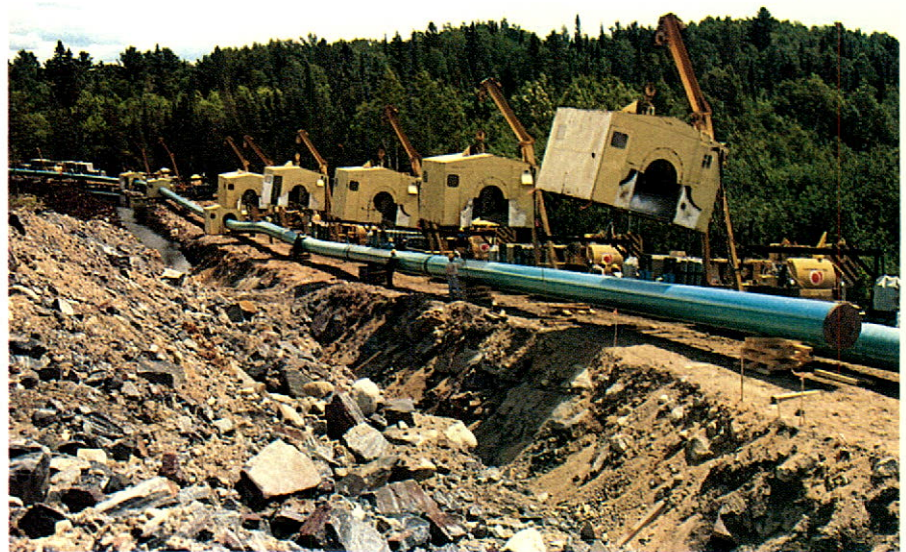
Automatic Welding Shelters being placed over pipe.
