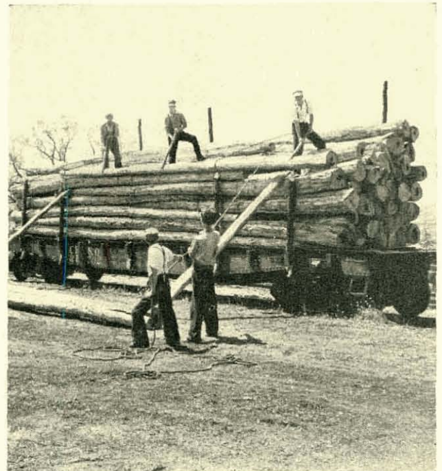
Unloading poles that will be used in the building of rural lines.
