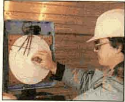
Viking sales meter station (above) is among the facilities monitored by NOVA's new gas control centre in Edmonton (left).
