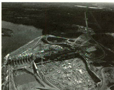
Construction site of La Grande-1
