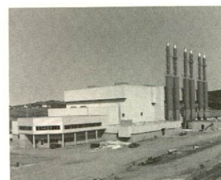
New diesel generating station on the Îles-de-la-Madeleine
