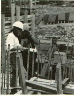
Inspecting construction work at La Grande-1
