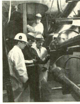
Visual inspection of underground installations
