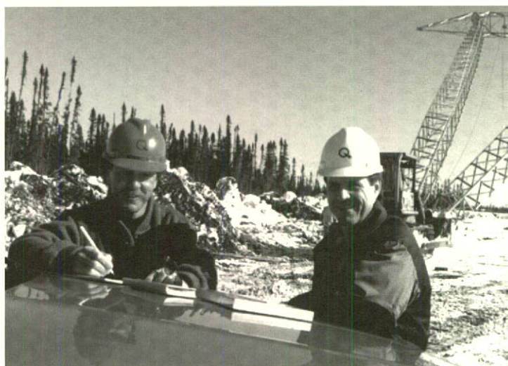
Building the 12th transmission line, near Chibougamau in northern Québec.
