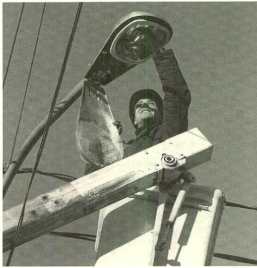
Installing a sodium luminaire in Greenfield Park, near Montréal.
