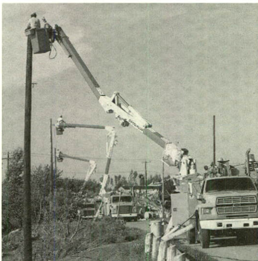
Working on the distribution system to improve service quality.
