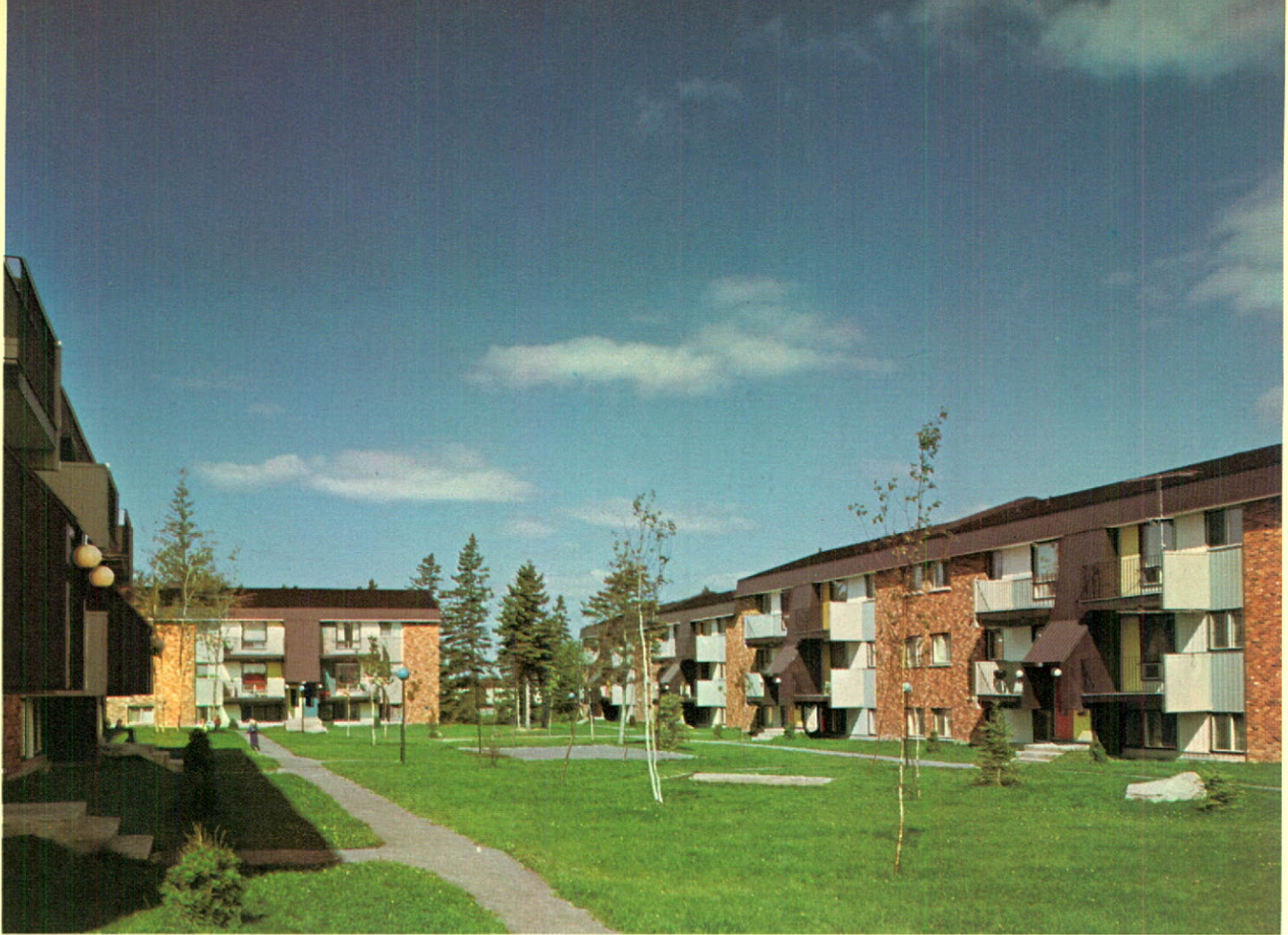
An all-electric housing development
