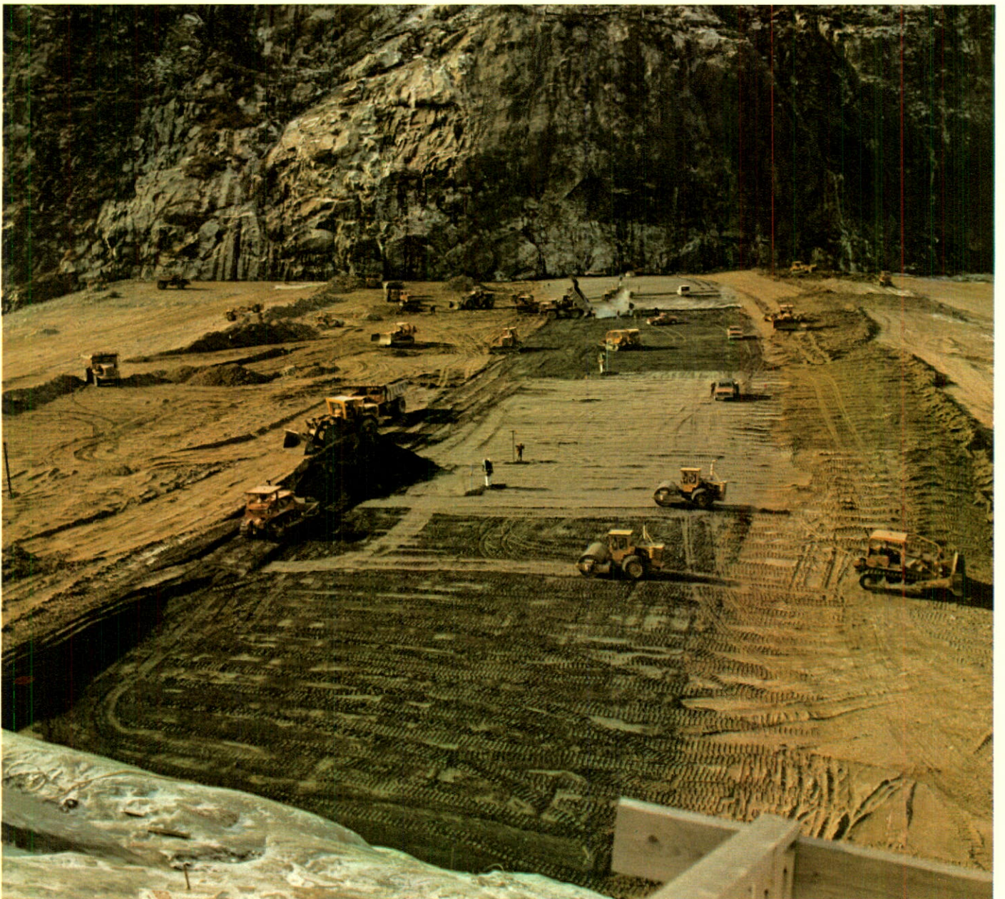
Manic 3: main dam under construction
