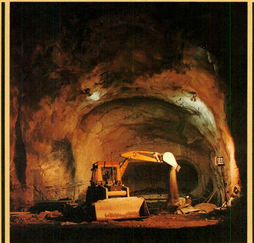
Excavation work, James Bay site.
