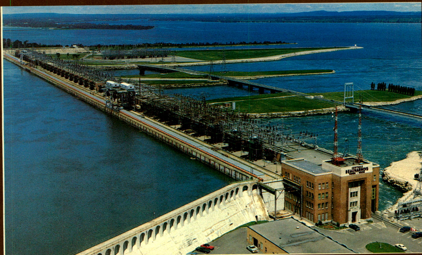
Beauharnois General view of the power station.
