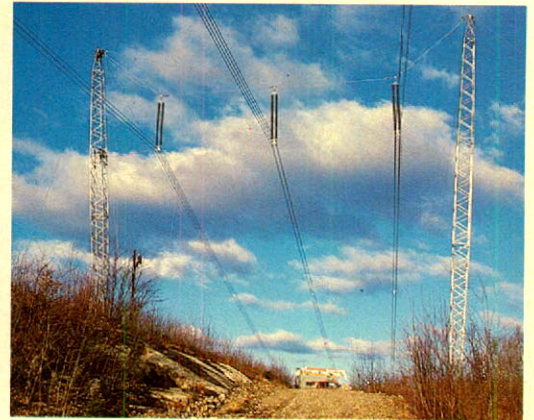
Hydro-Québec's new chainette (cross-rope) tower.
