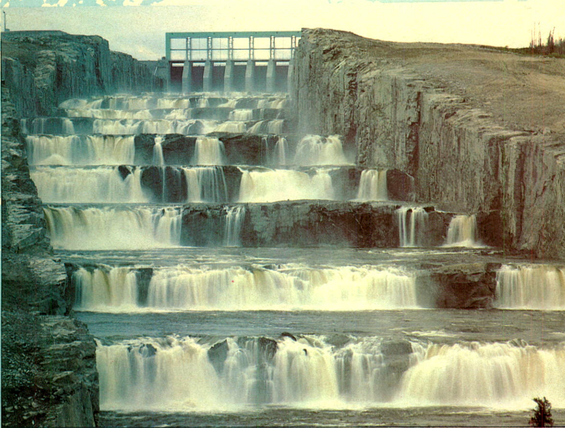
The LG-2 spillway.
