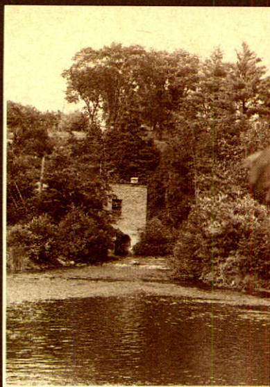
Les Cèdres power station under construction in 1912.
