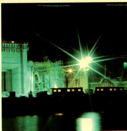
LG 3 construction site.
