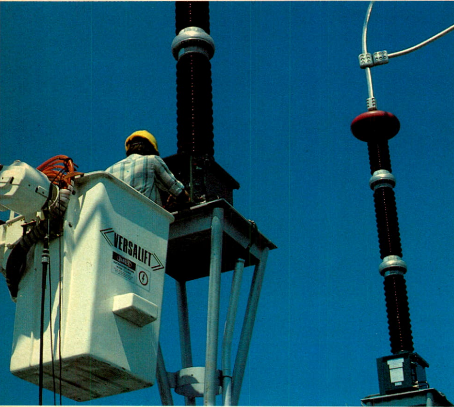
Construction of Hertel substation.
