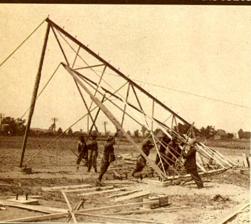
Erection of a transmission-line tower in the 1920s.
