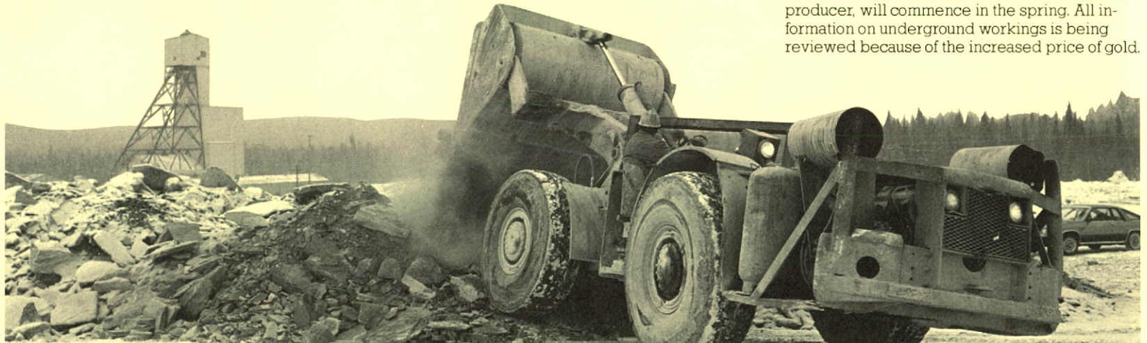
Load Hall Dump Machine dumping a load near the headframe at Mine de Bousquet, Quebec.
