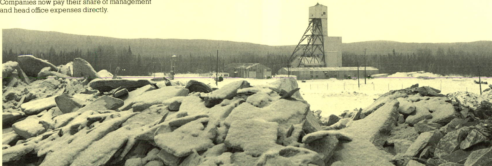
Headframe at Mine de Bousquet, Quebec.
