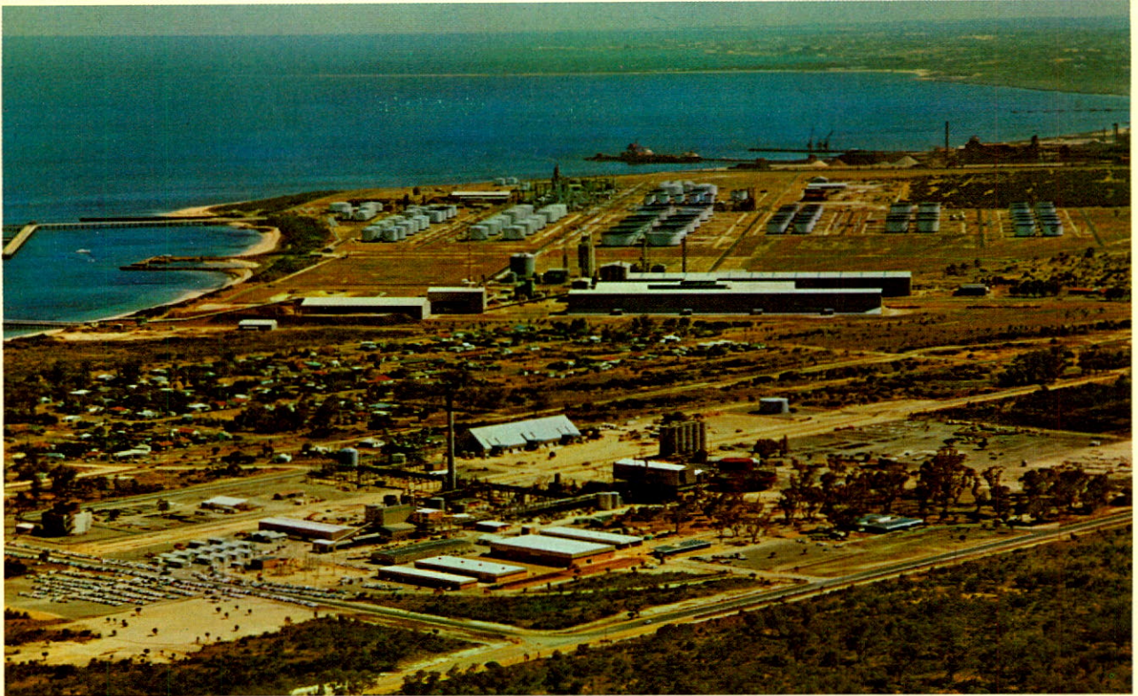
NICKEL REFINERY (FOREGROUND) OF WESTERN MINING CORPORATION LIMITED AT KWINANNA, WESTERN AUSTRALIA
