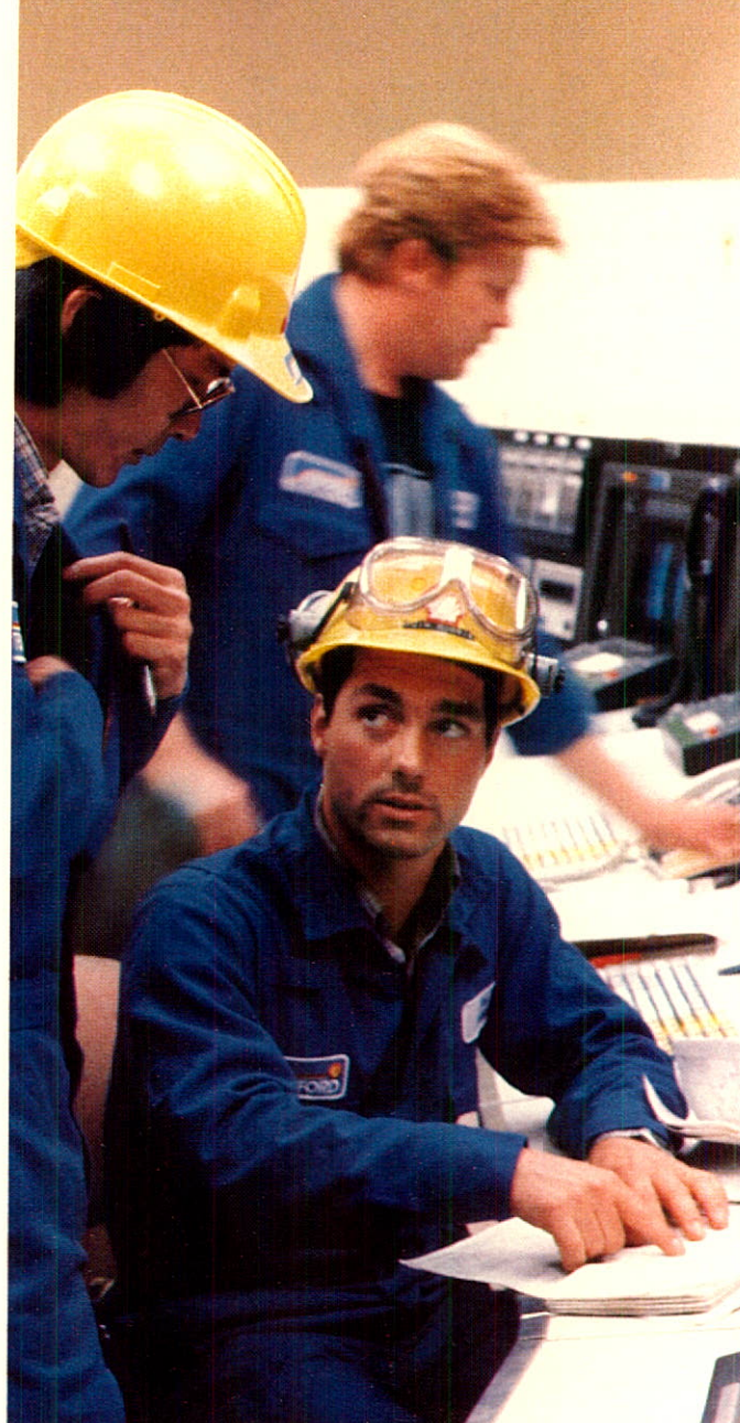
Team members Jim Dobbie (seated), Mike Lim (foreground) and Erick Bennett in one of two micro-computer centres from where operations are monitored and controlled at the new Scotford refinery in Alberta.
