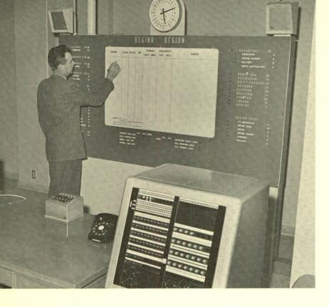
In Regina's Network Management Center, the staff can take action to avoid serious congestion and blockage of long distance calls. The display panel and supervisory cabinet are two of the tools used to indicate and correct overload conditions.
