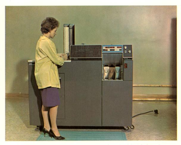
New methods of billing customer's long distance accounts have been adopted by Saskatchewan Government Telephones. Made necessary by the introduction of Direct Distance Dialing, the Corporation's Data Processing Centre can also handle "mark sense" tickets from manually operated offices.
