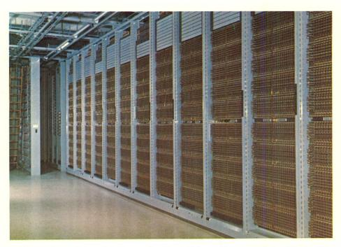
Highly complex equipment is necessary for Direct Distance Dialing now being introduced in Saskatchewan. Hundreds of crossbar switches (like those above) located in major SGT exchanges, will be scanned to find an idle route to the called telephone. The numbers dialed are stored in the sender (below) and the caller's own number is verified through intricate cross connections (shown on the cover).
