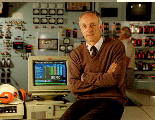
By combining the best features of all the efficiency monitoring systems NSPC tested, Peter Whitehouse and Kevin MacDonald created the ideal "custom" system for the Corporation. Peter is pictured in his lab at Trenton Generating Station.
