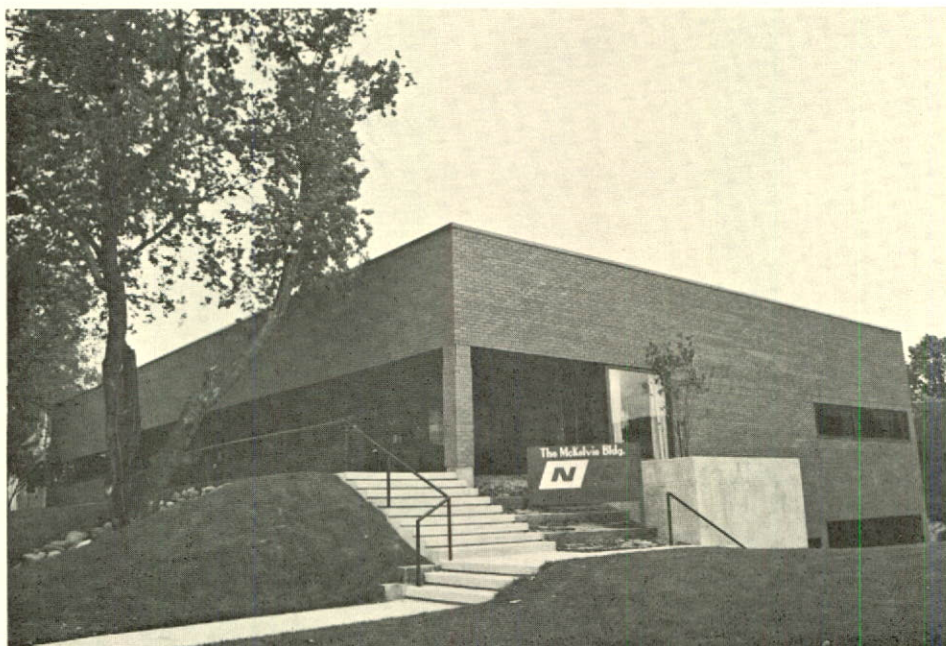
Northern Telephone's Head Office, "The McKelvie Building", located in New Liskeard, named in honour of Donald McKelvie, former President and Past Chairman of the Board, who served the Company for 47 years.
