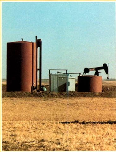
Pump and Storage Facilities at Keho 6-10.
