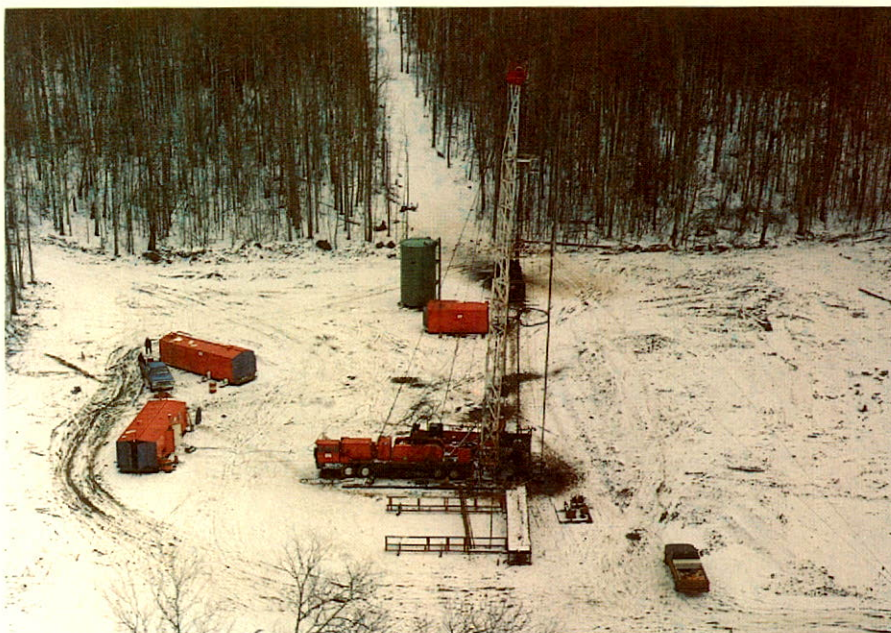
Service rig completing Otter 12-9.
