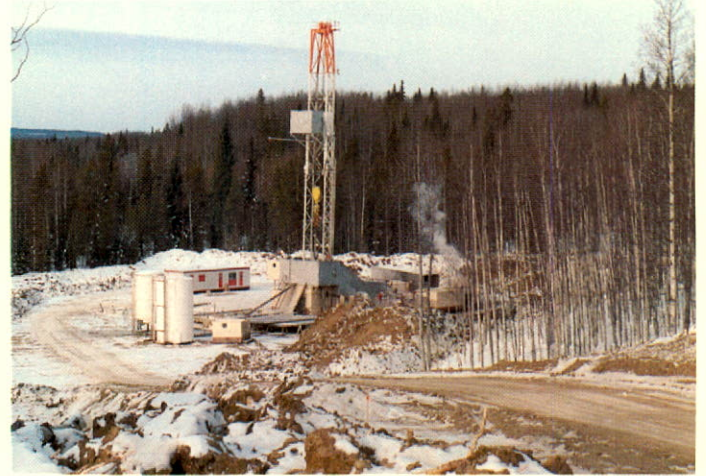
Drilling of a new well
