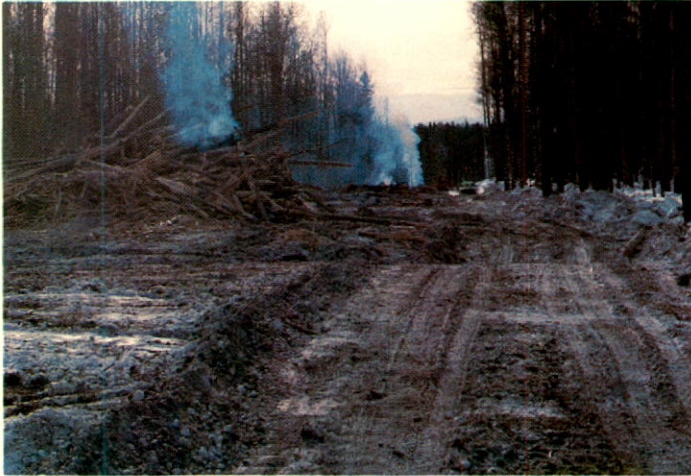
Building a road to a new location
