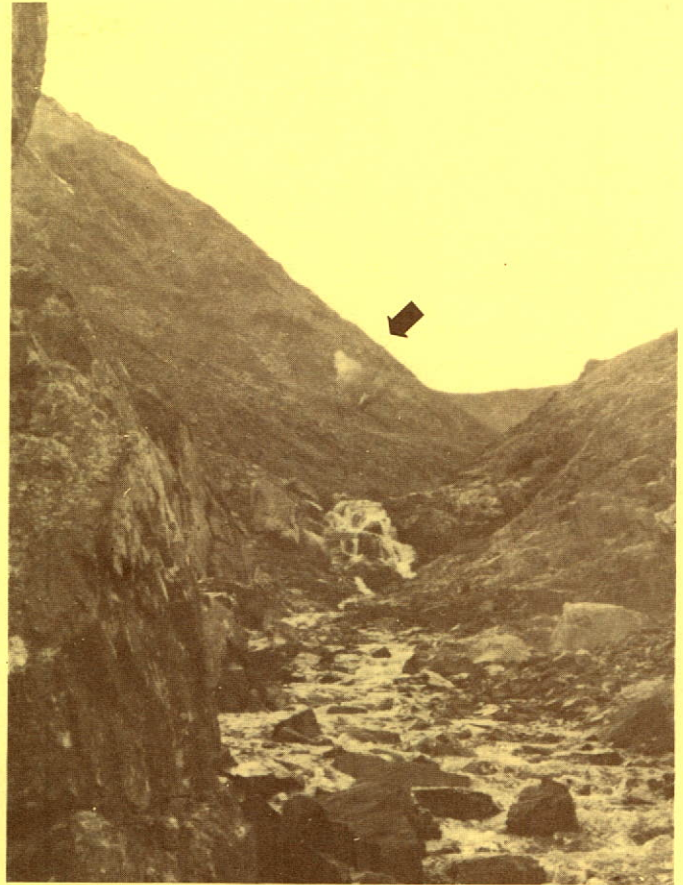
BLASTING ON #1 SHOWING
