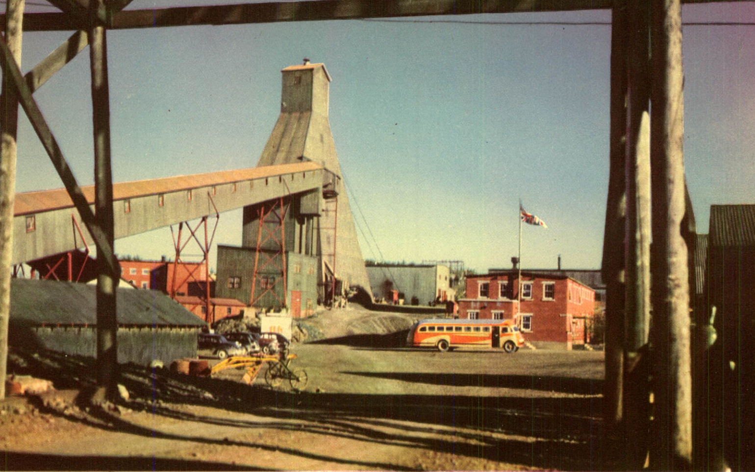
HEAD FRAME AND BUILDINGS AT "A" SHAFT WAITE AMULET MINES, LIMITED
