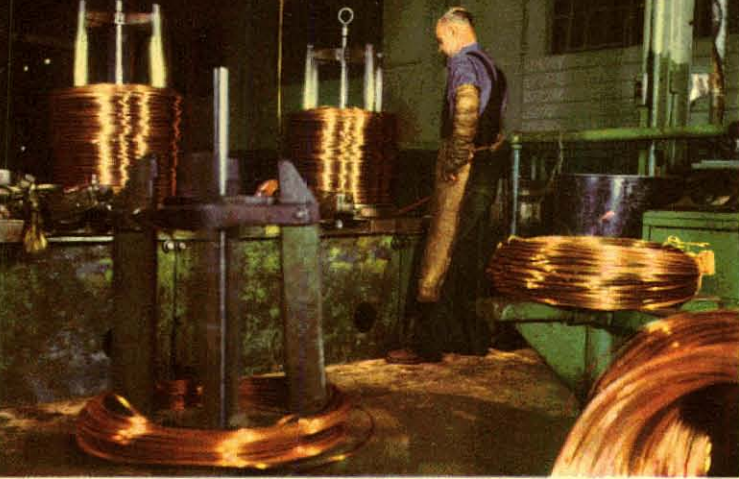
DRAWING WIRE AT CANADA WIRE AND CABLE, LEASIDE
