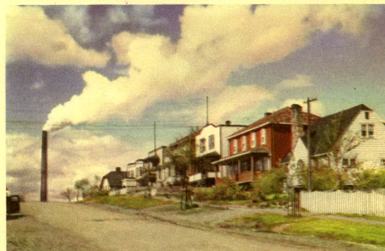
TYPICAL OWNER OCCUPIED HOUSES
