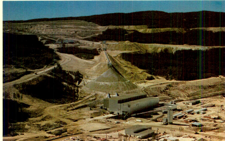
Lornex, the copper-molybdenum mine in British Columbia's Highland Valley, began production in 1972. Overall view shows the plant and related facilities in foreground, the coarse ore stockpile and conveyor from the primary crusher, and in the upper left, the production pit.
