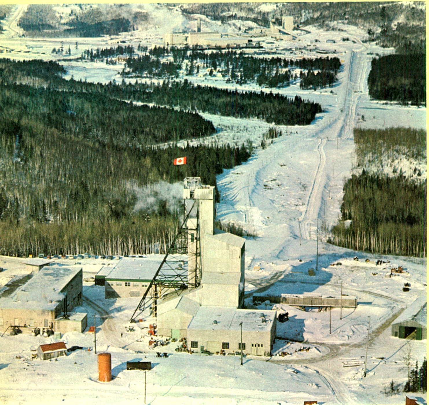
Winter view of New Quirke, in foreground, and the Quirke mill. Construction of a semi-automatic, ore-hauling electric train line connecting the mine and mill began last year. The line is designed to move 200 tons of ore per trip in 13 cars, each with a 15-ton capacity.
