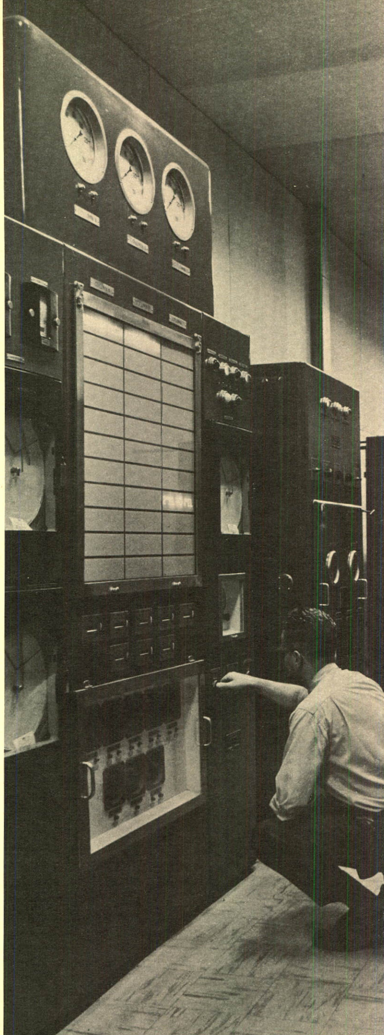
Ion exchange control unit for the production of uranium oxide at the Nordic mill, Elliot Lake, Ontario.
