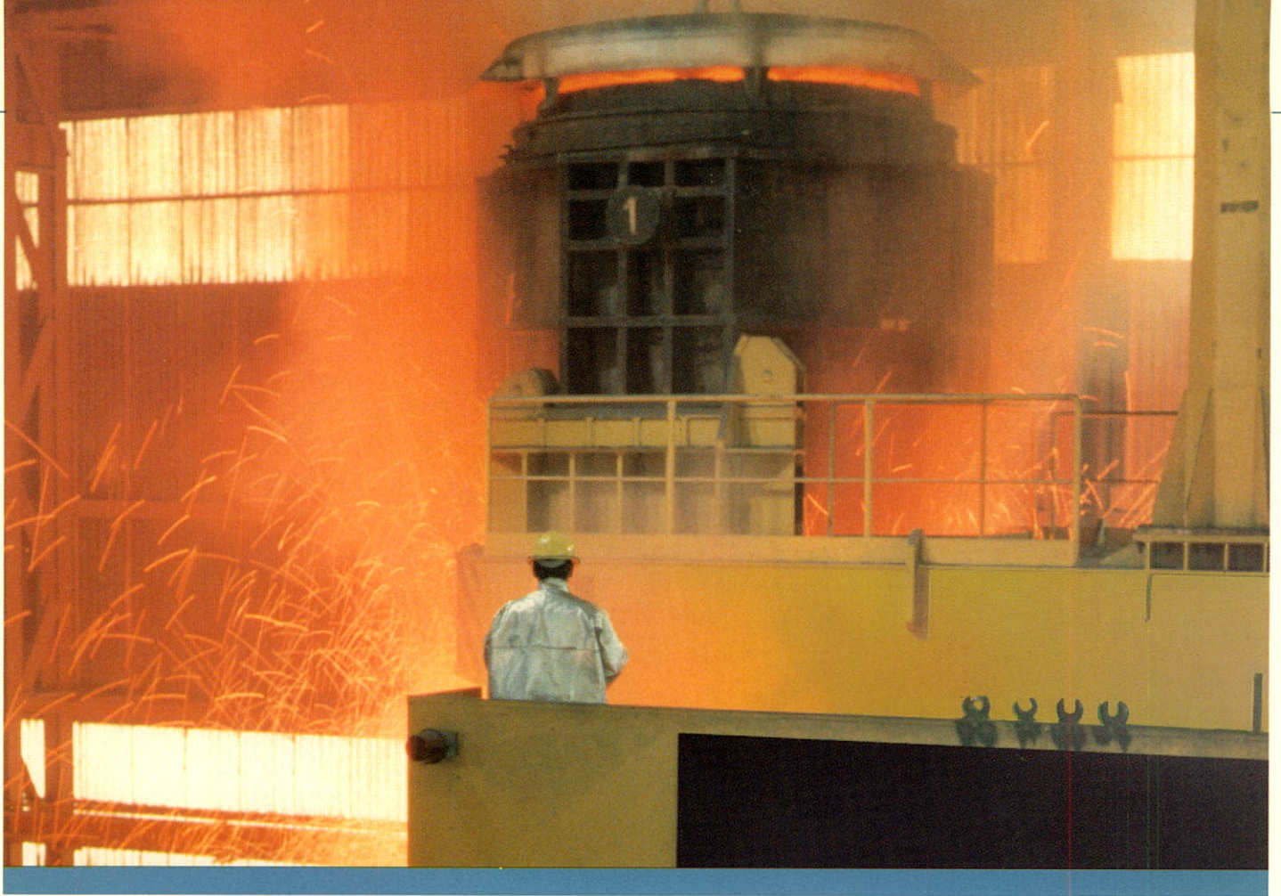
The new continuous caster at Atlas Specialty Steels, Welland processes a wide range of billet products.
