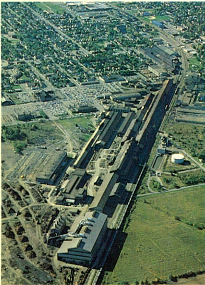
Atlas Steels' Welland plant. New $4.1 million facility seen at right, purifies and recycles plant cooling water. Steel going up to the left of main plant is part of $11 million expansion of the cold bar finishing operation, scheduled for completion in 1982.
