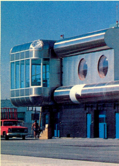
Stainless steel for Lethbridge's gleaming new $4-million airport terminal building came from Atlas Alloys. Stainless is finding increasing use in the construction field generally.
