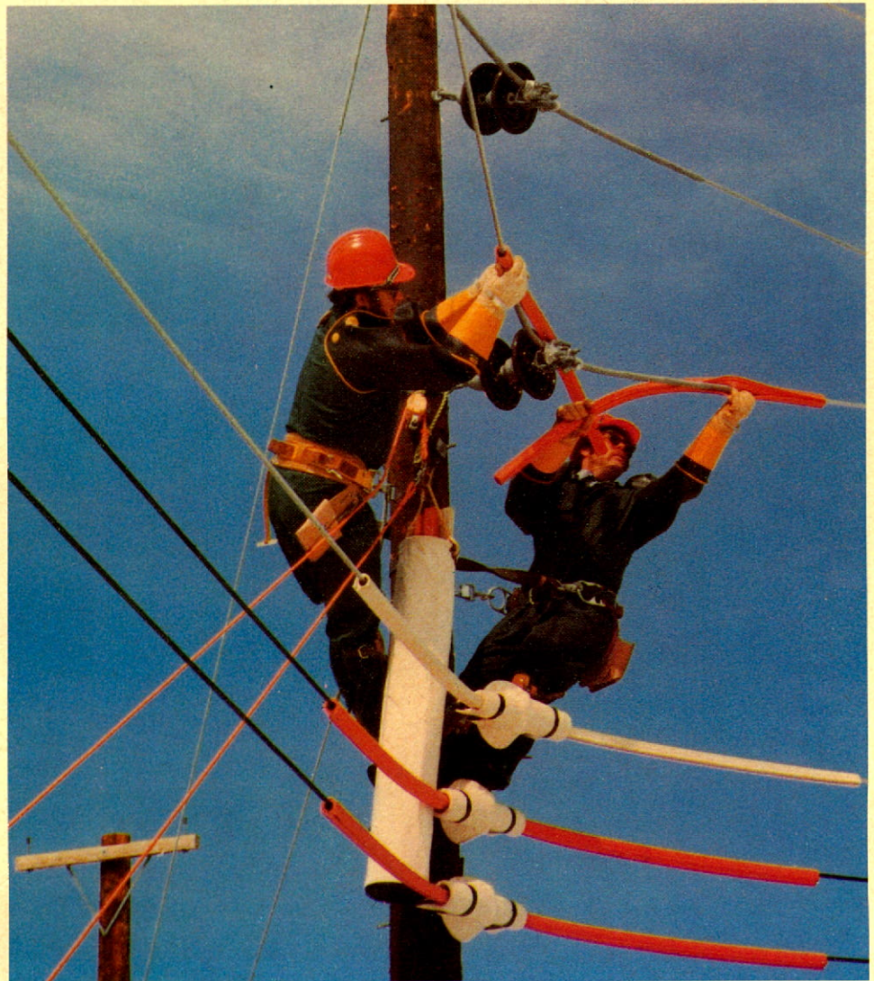
Employees carrying out hot-line work on a PDD distribution line.
