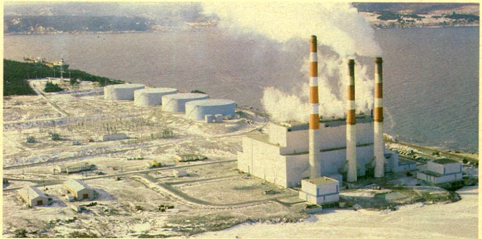
Hydro's 450 megawatt thermal generating station at Holyrood.
