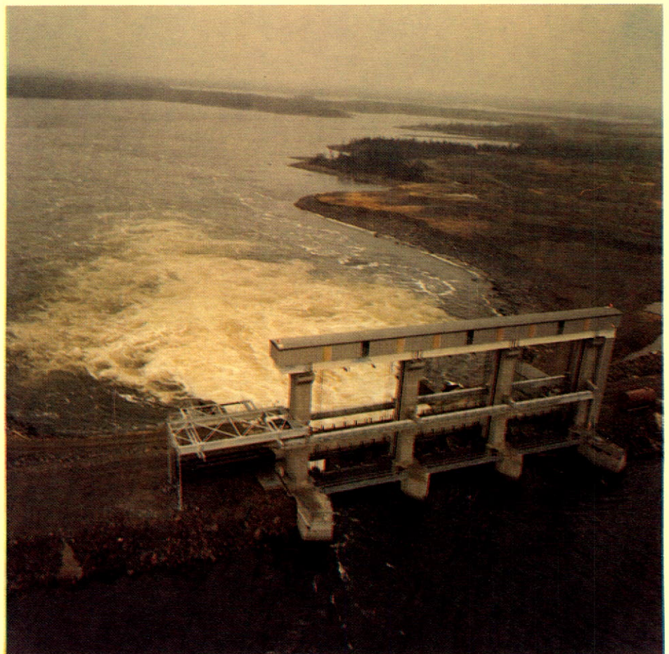
Lobstick — Main Control Structure in the Churchill Falls hydro-electric development.
