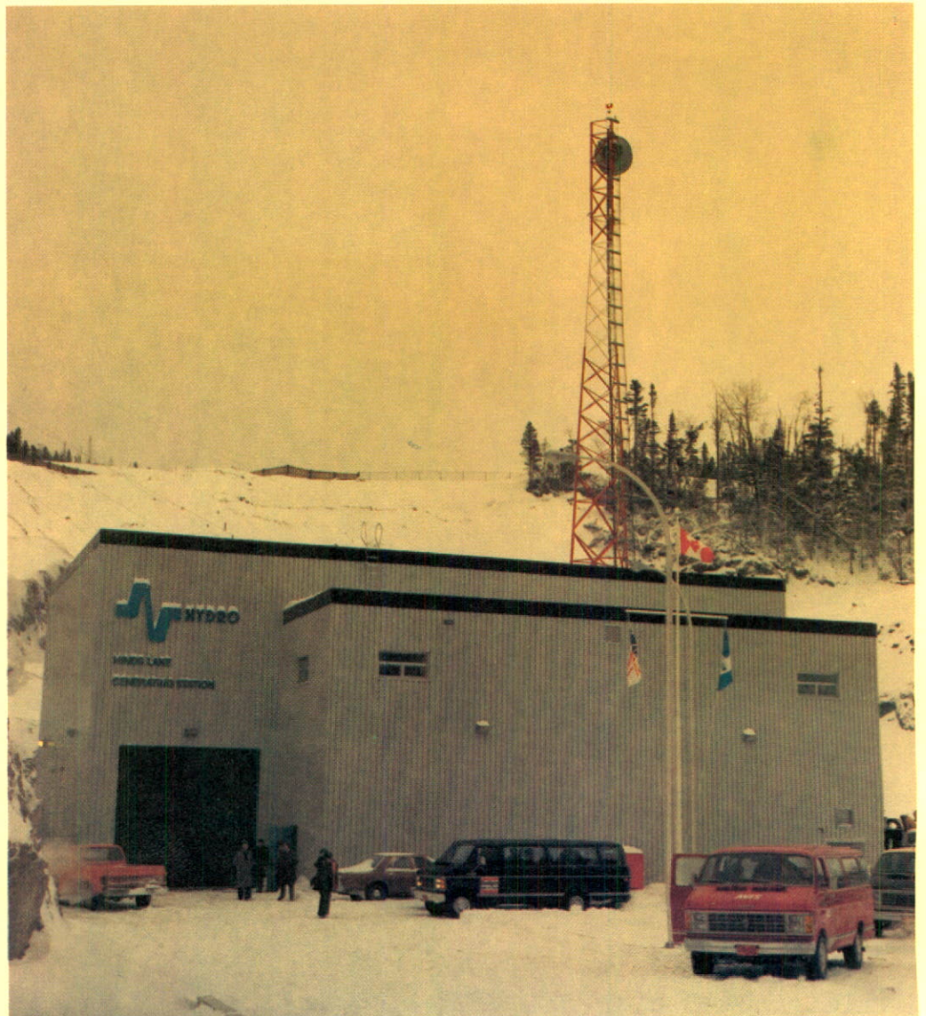
75,000 KW Hinds Lake hydro-electric generating station was officially opened on December 17, 1980. Located on the West Coast of the Island of Newfoundland the plant was built at a cost of $84.7 million.
