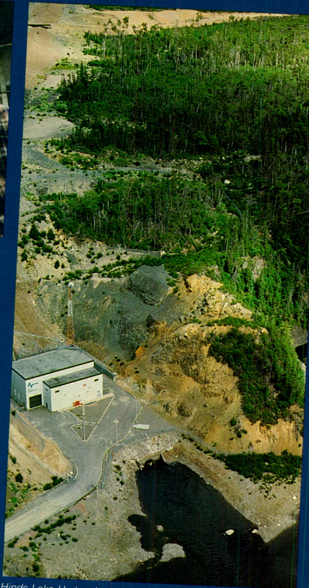
Hinds Lake Hydro-electric Generating Plant
