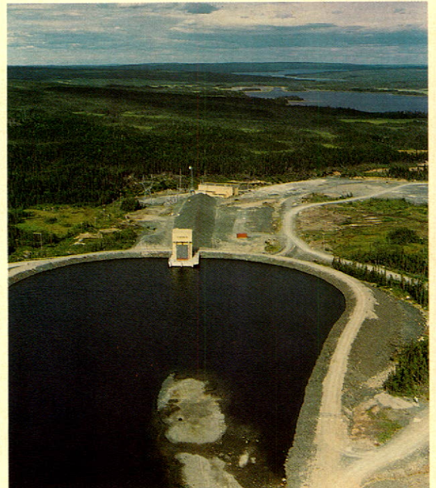
Forebay of the Upper Salmon Hydro-electric Generating Plant
