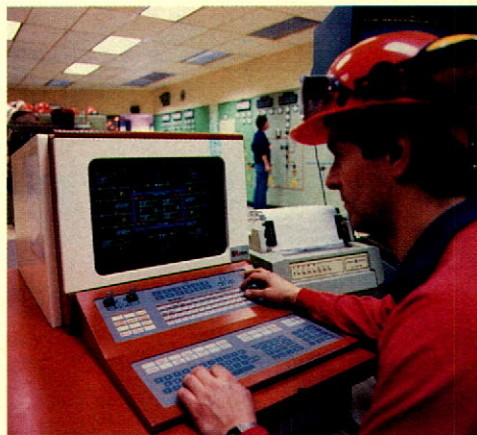
Thermal Plant Operator
