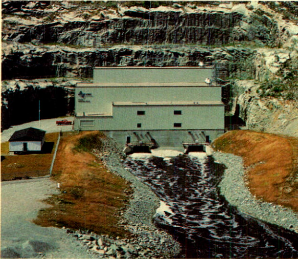
Cat Arm Hydro-electric Generating Plant
