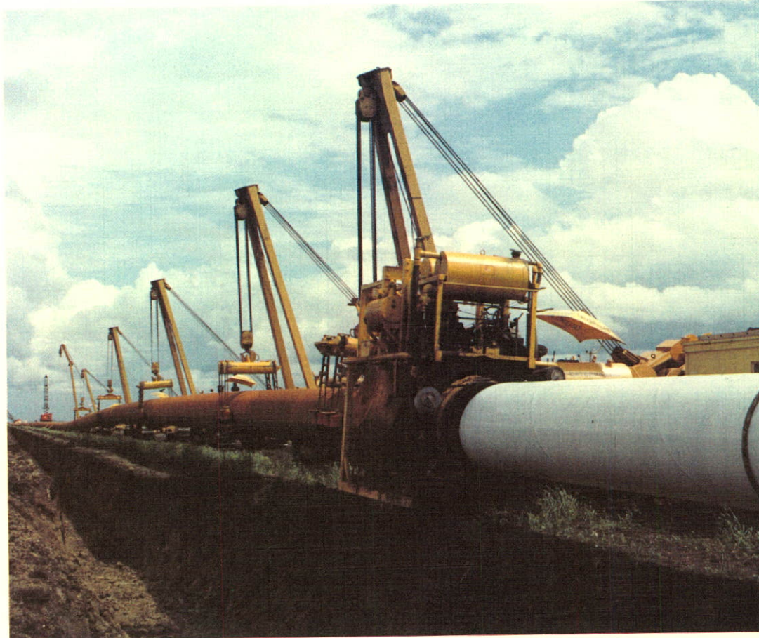
TransCanada PipeLines lays 48-inch pipe near Portage La Prairie, Manitoba in summer, 1981.
