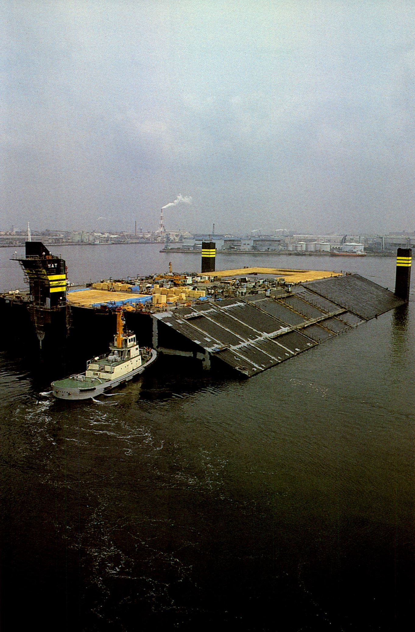
The MAT, at completion of construction at Hitachi Zosen Shipyard in Japan.
