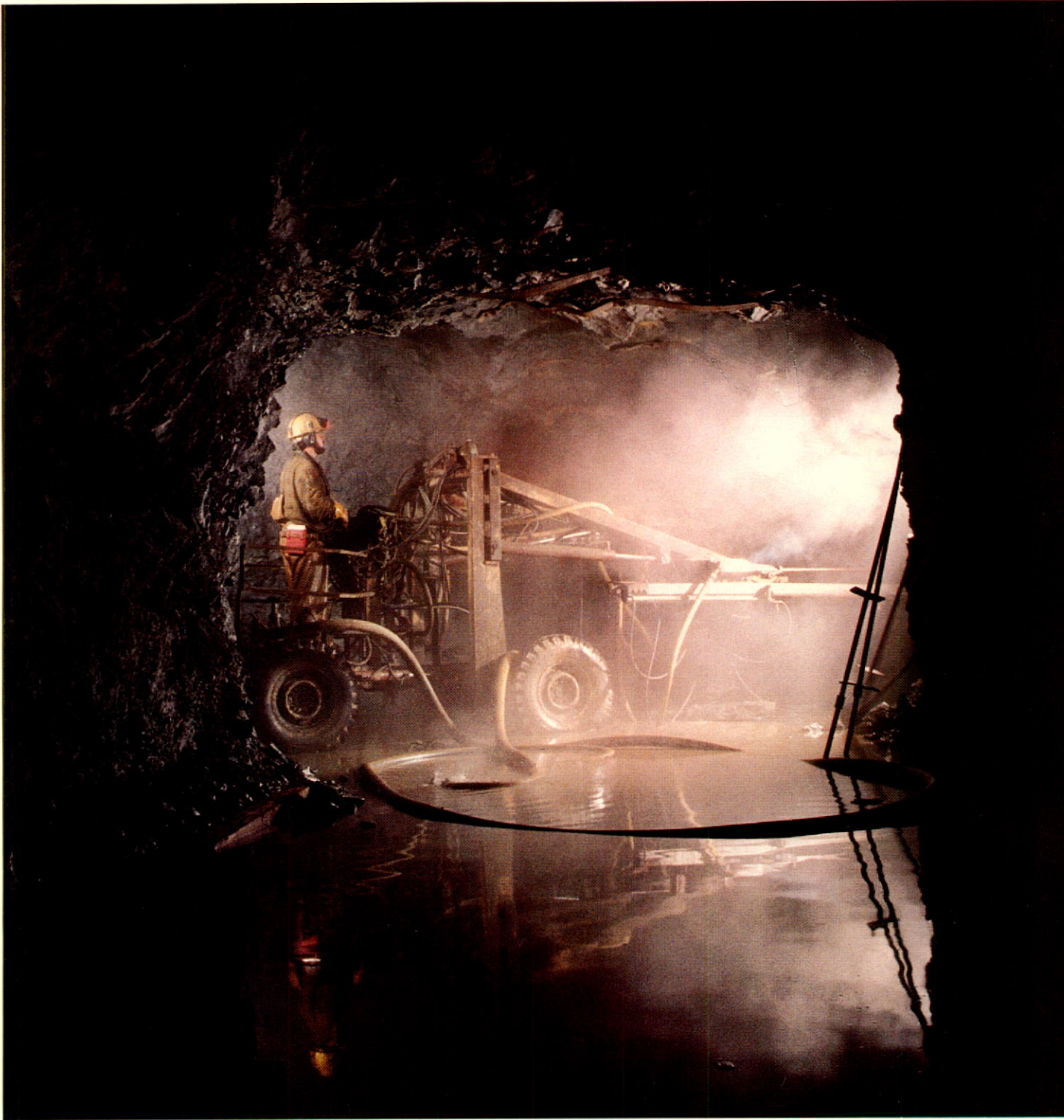
Drill jumbo at the Dome Mine
