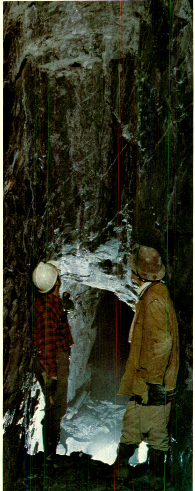
Mine supervisors examining a shrinkage stope at Campbell.
