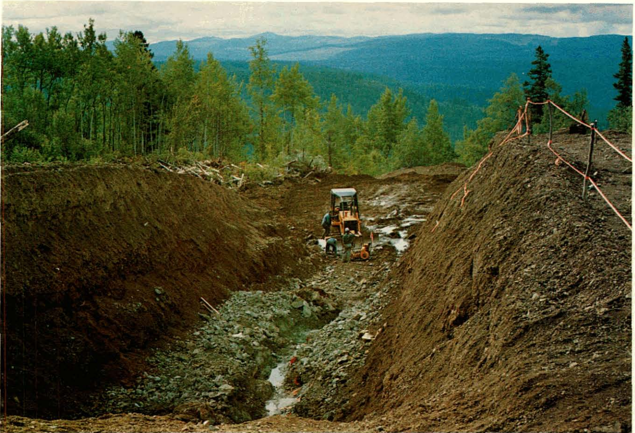
Trench exposing bedrock at a gold prospect in the Quesnel River area of B.C.
