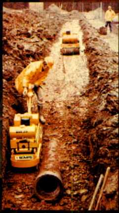
Koehring Company was acquired in 1980. Workman (right) makes final adjustments on large hydraulic excavator at Milwaukee plant. Inset (above) shows a walk-behind BOMAG vibratory roller used for stabilizing and smoothing soil in newly dug trench. See Pages 34-35 for introduction to Koehring.
