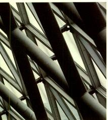
The higher strength-to-weight ratio of hollow structural sections allows designers to specify sections which are lighter in weight and smaller in size to carry the same load.
