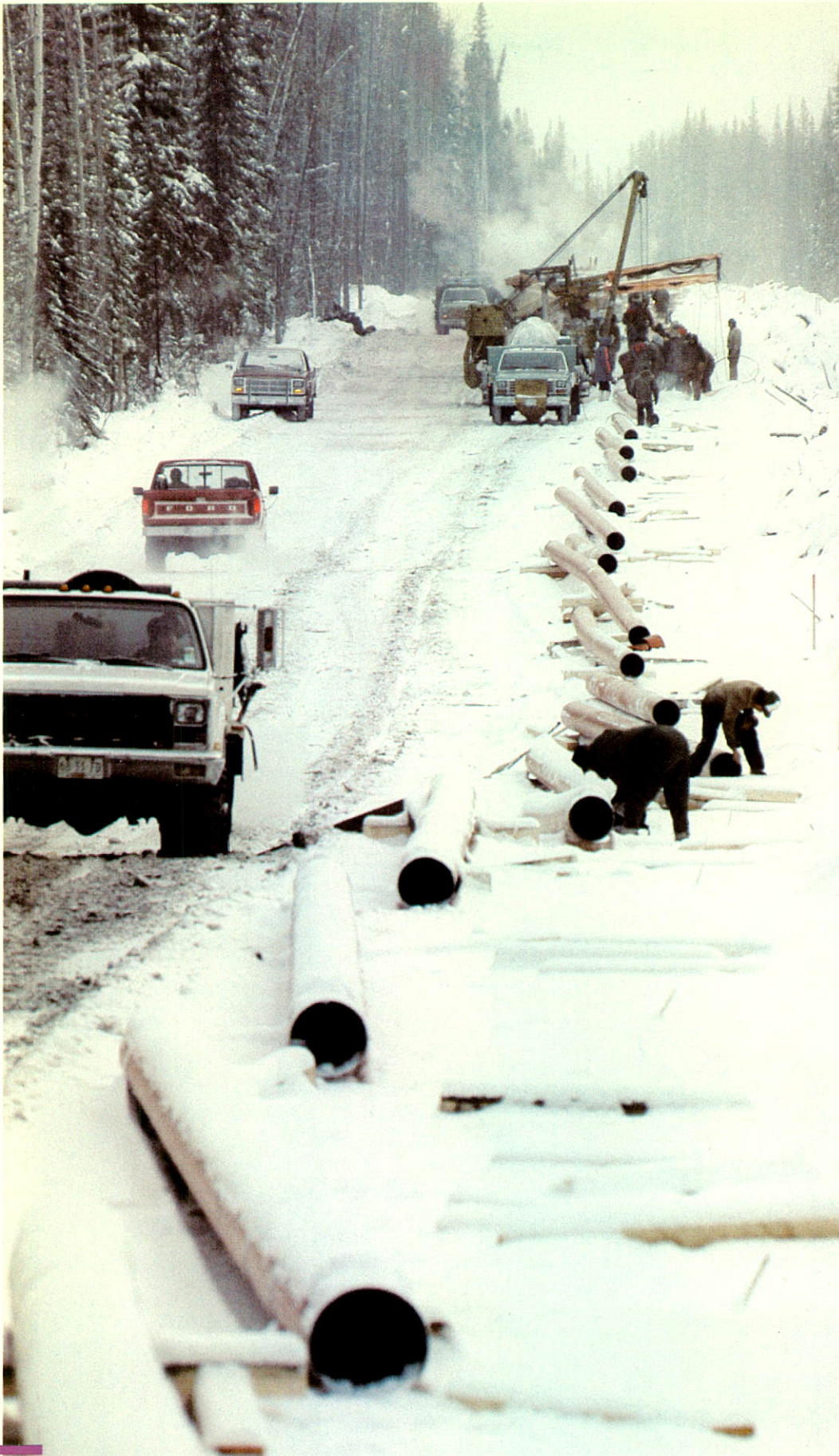
Arctic ditching machine cuts through permafrost as seen in wall of the ditch. A view along the right-of-way shows sections of pipe being positioned for the welding team. Hugh Sangster, Assistant Project Manager, reviews progress with Brian Thomas at Fort Simpson.
