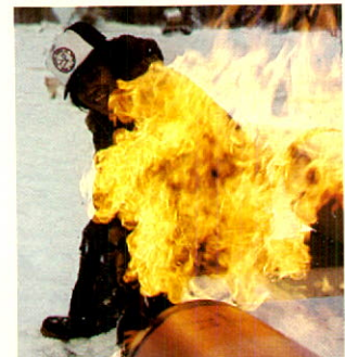
Welding team joins pipe sections. Prior to welding, the pipe ends are heated by propane torch in -35°C weather.
