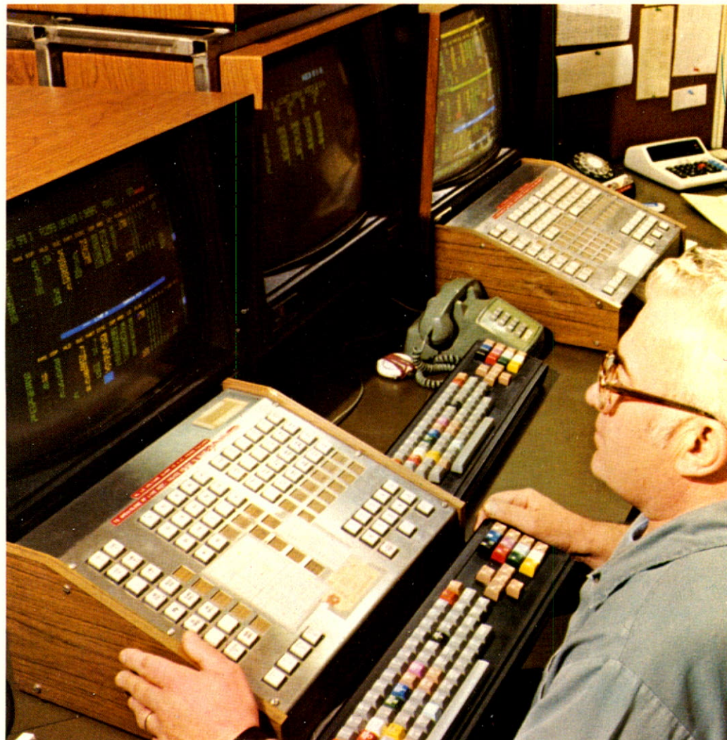
Remote control centre at Sarnia.
