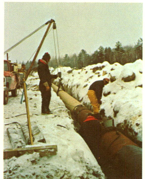
Lowering in 30" pipe under winter conditions.
