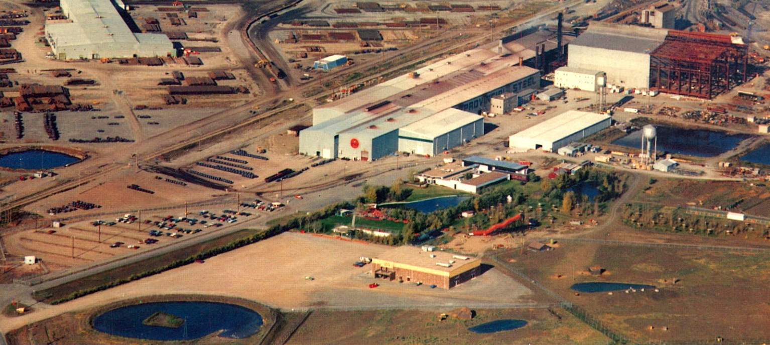
▲ A recent aerial view of the Ipsco Regina plant showing the expanded facilities.
