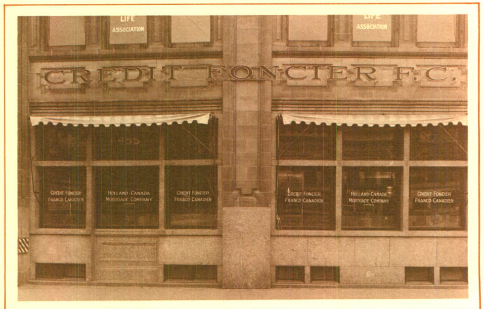
During the depression, Credit Foncier acquired the Holland-Canada Mortgage Company
