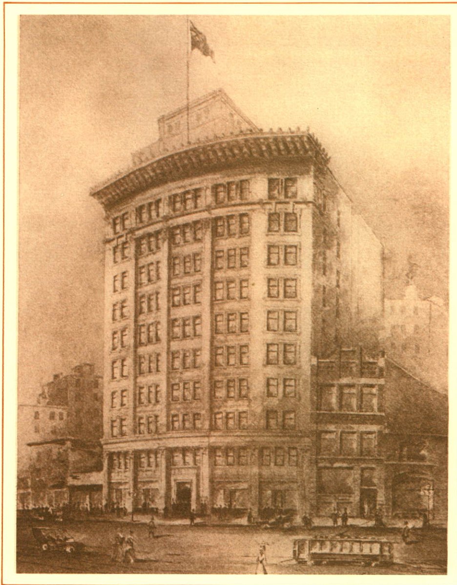
Confederation Life Building
