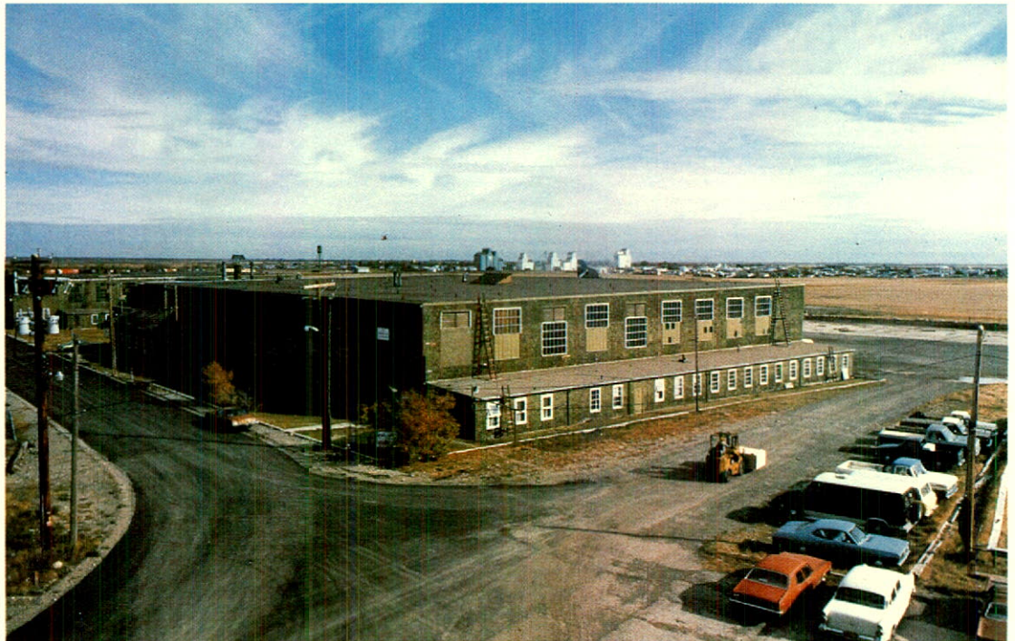
Top. Fort Macleod Plywood Plant. Bottom. Creston Sawmill.
