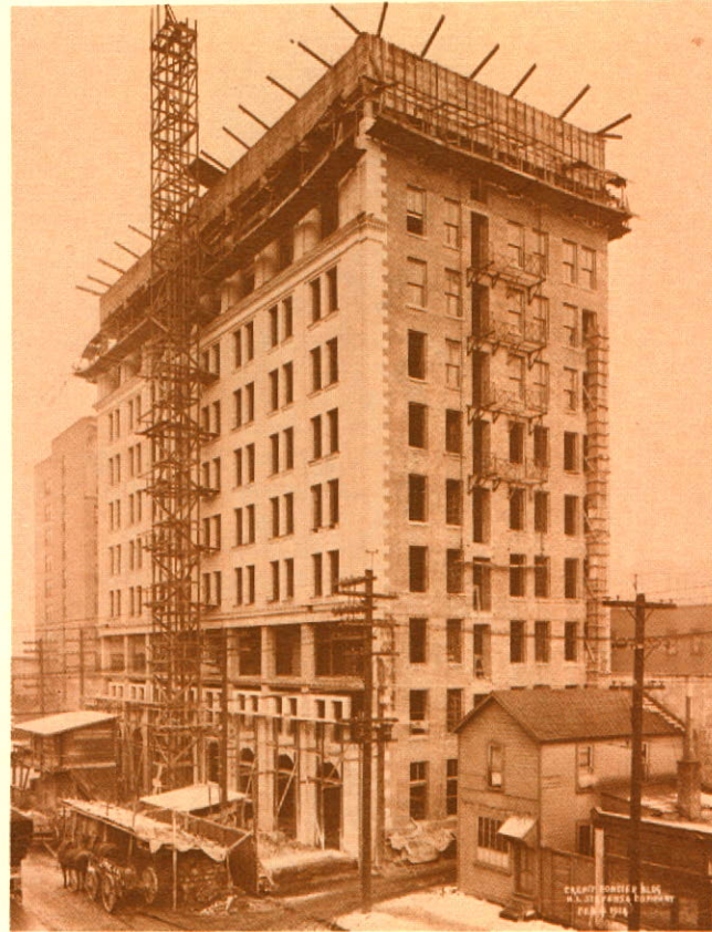
Our Vancouver office building under construction in 1914
