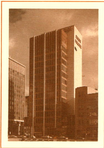
Present head office building
