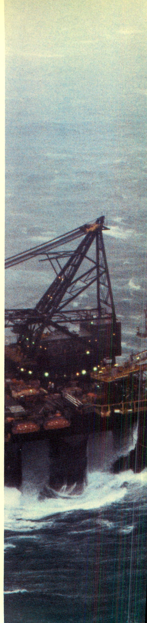
The South Brae production platform is 648 feet tall, weighs 55,000 tons, has four acres of deck space, and provides living accommodation for 240 people. The derrick barge on the left will be moved off location in late 1983.
