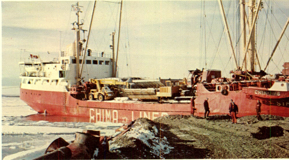
First vessel to arrive and discharge at the newly constructed pier at Resolute Bay, August 1972.
