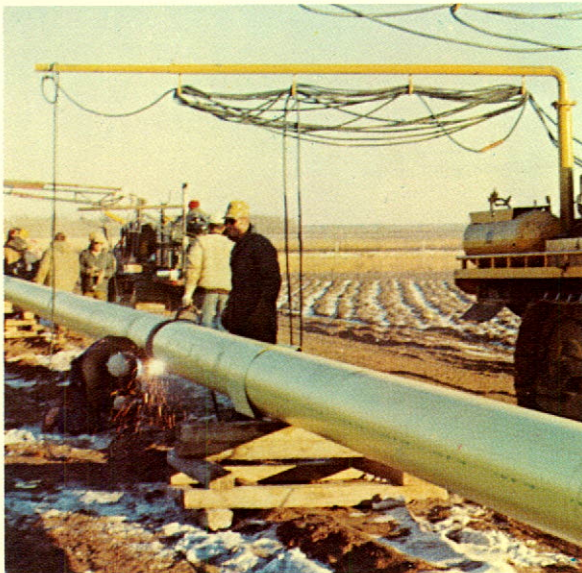
Wonderly & Kershaw constructing a pipeline in Alberta.
